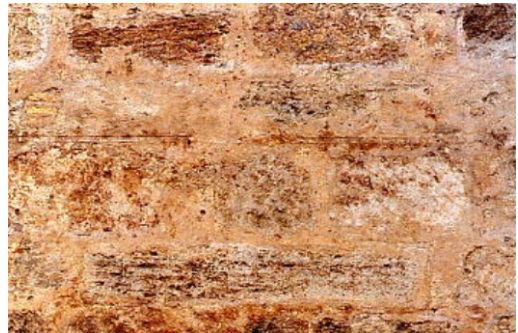
Exterior ornamental cover at the Temple Church. Feigned ashlars over ashlars.
