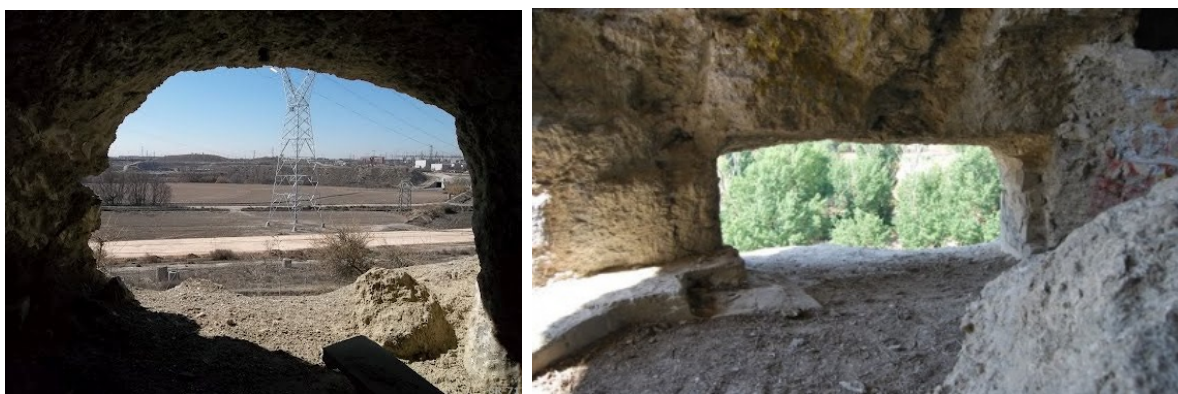
Figure 10. Perforations in horizontal galleries, by way of loopholes.
