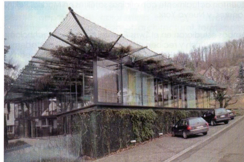
3, 4 - Ricola sales Building, Herzog & de Meuron, Oberwil (Switzerland), 1979-1980 in http://www.flickr.com/photos/10230887@N02/1479794325/
