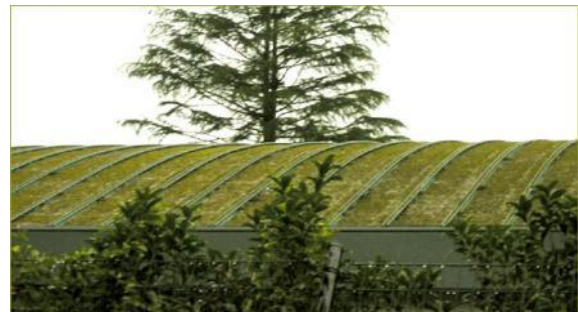
Figure 1 Moss Catch. Roof
