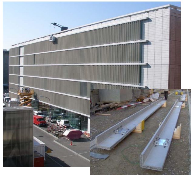
Figure 1 – Application of CFRP prestressed concrete L-shaped beams for structural façade elements in Zurich, Switzerland [1].
