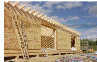
Figure 1. Example of straw-bale construction of load-bearing wall. [1]
