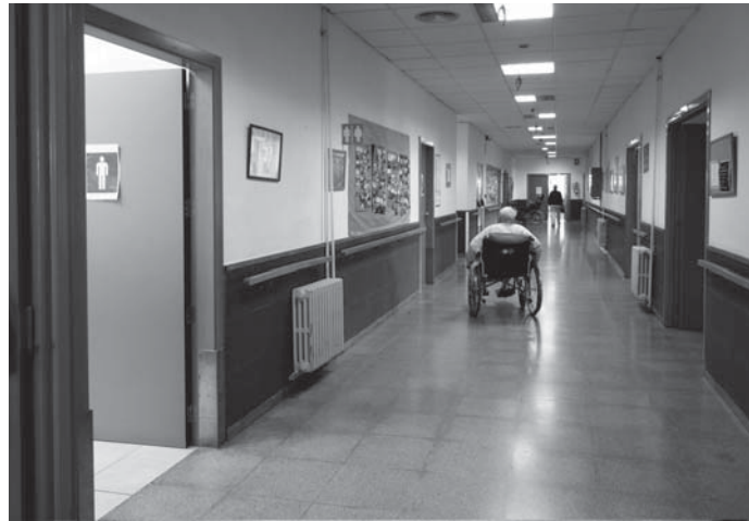
Fig. 6. Interior of El Pinar de Castellón Residence. Current state. Hallway
