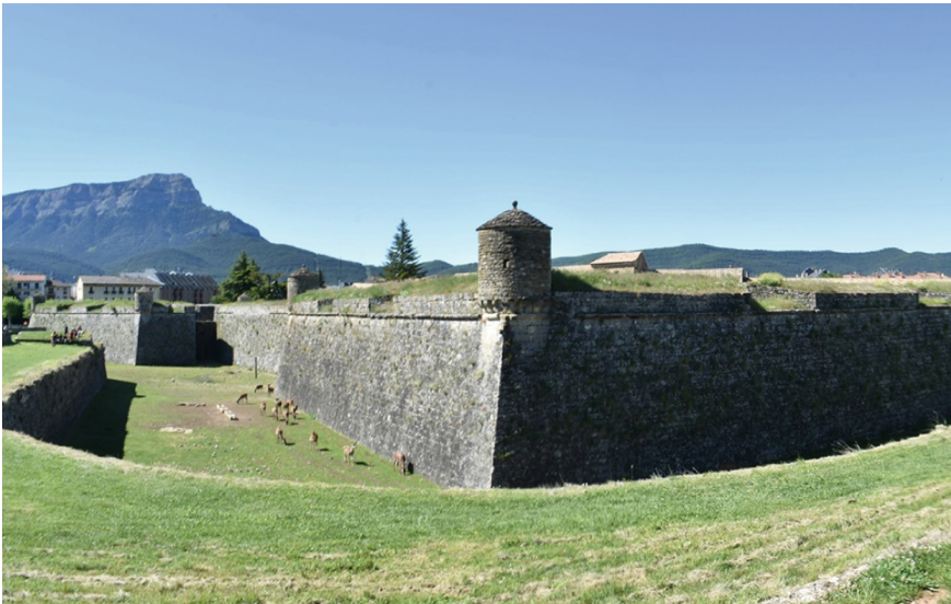
Fig. 8. Northeast bastion of the San Pedro Castle in Jaca. 2019. Photo by the author.
