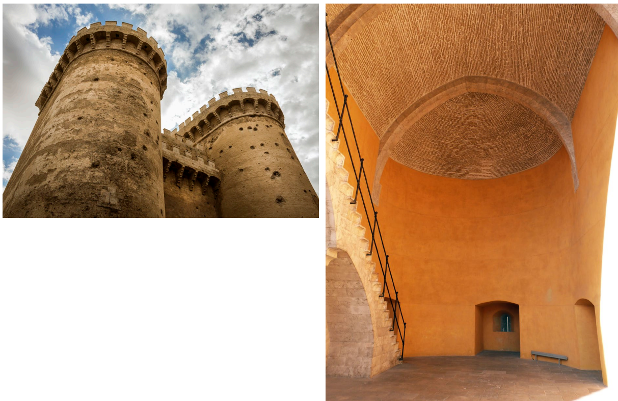
Figura 3. Restoration of the original colors of the Torres de Quart, the gates belonging to the medieval wall of Valencia. GICA-UPV together with Javier Benlloch Marco and Manuel Jesús Ramírez Blanco Architects, 2007.
