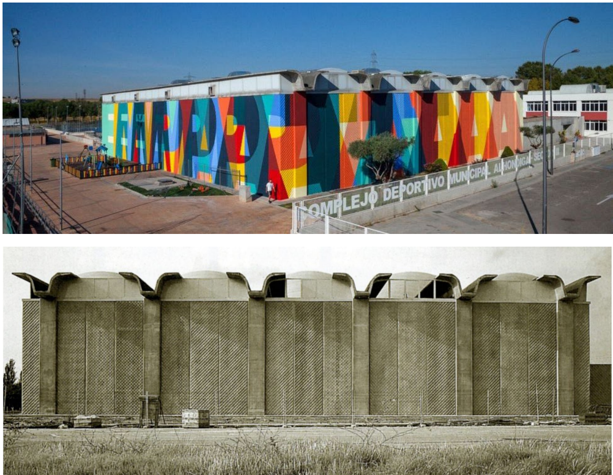
Figure 1. The Alhóndiga Sports Center in Getafe, work by architect Miguel Fisac. Above: Original appearance in 2004. Below: Appearance after Boa Mistura's intervention, at the festival organized by Cultura Inquieta. Source: El País Digital. https://elpais.com/cultura/2020-09-25/los-coautores-del-edificio-de-fisac-exigen-a-alcaldesa-de-getafe-que-limpie-las-pintadas-de-boja-mistura-en-un-mes.html
