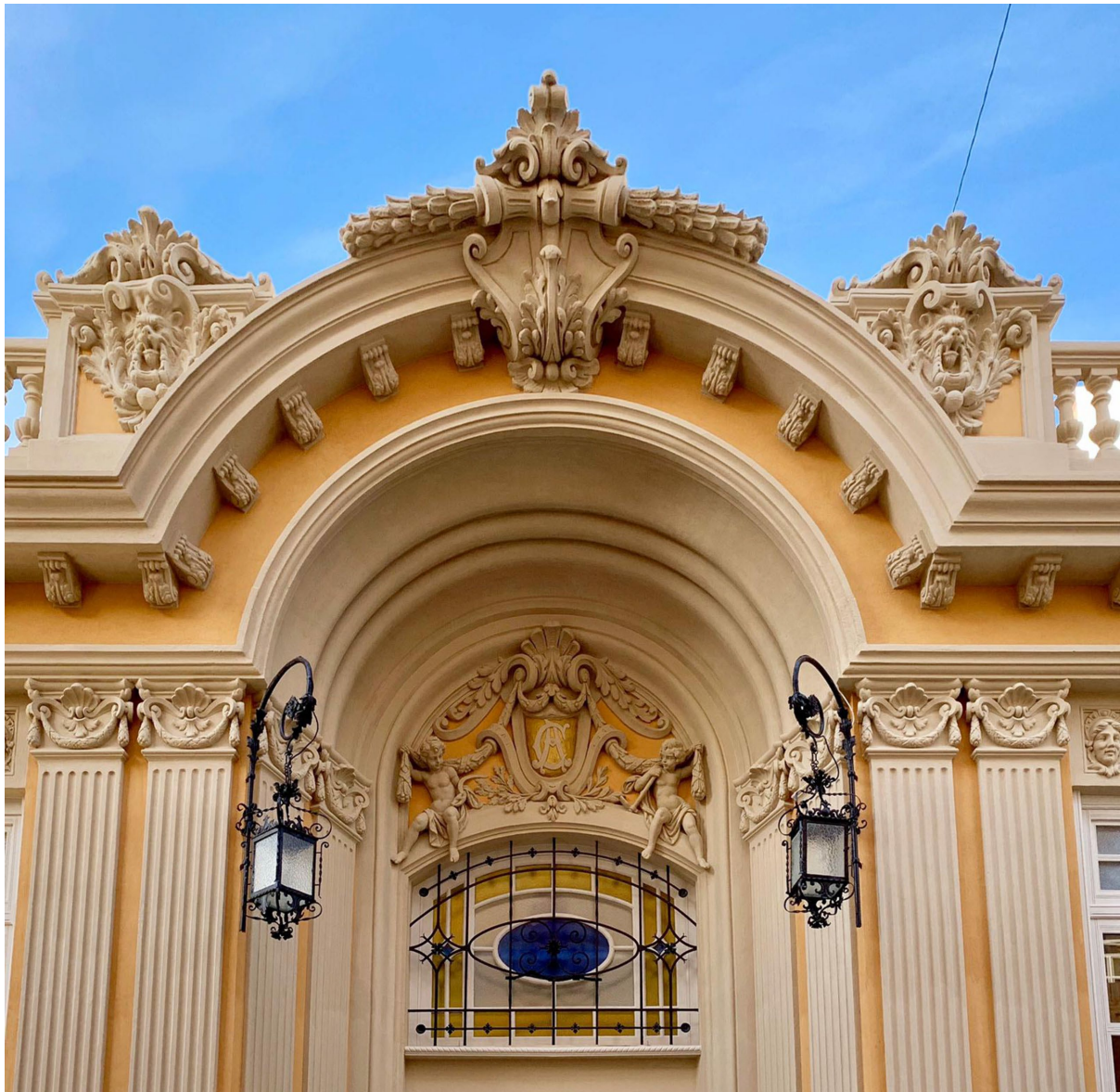
Figure 5. The traditional ocher colors in Valencian architecture were recovered in this eclecticist building belonging to the Rice Union in Alfafar, Valencia, 2018. GICA-UPV together with Javier Hidalgo Mora Architect. Source: https://grupocolor.webs.upv.es/?page_id=2764
